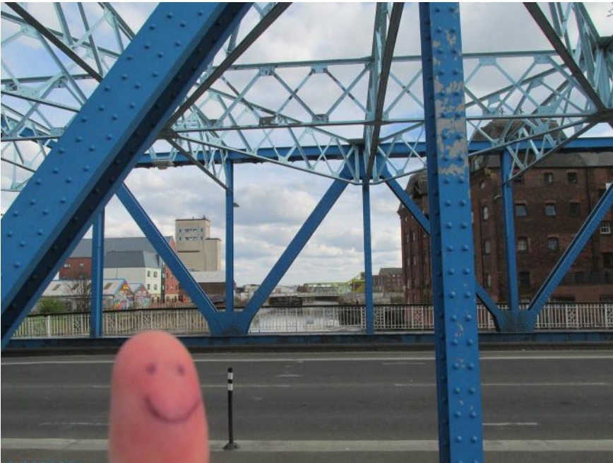
Crossing over the 'River Hull' into the city centre.
